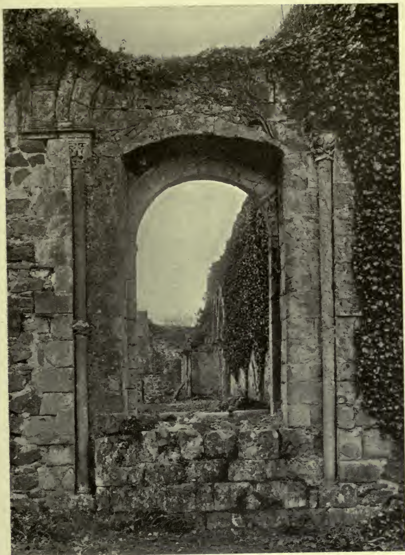
RERE-ARCH OF WEST PROCESSIONAL DOORWAY.
